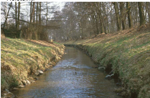
FIGURE 3.5: Clearly no reference site: the stream is scoured and the banks are fixed with stones (Rotbach, Lower Rhine area).
