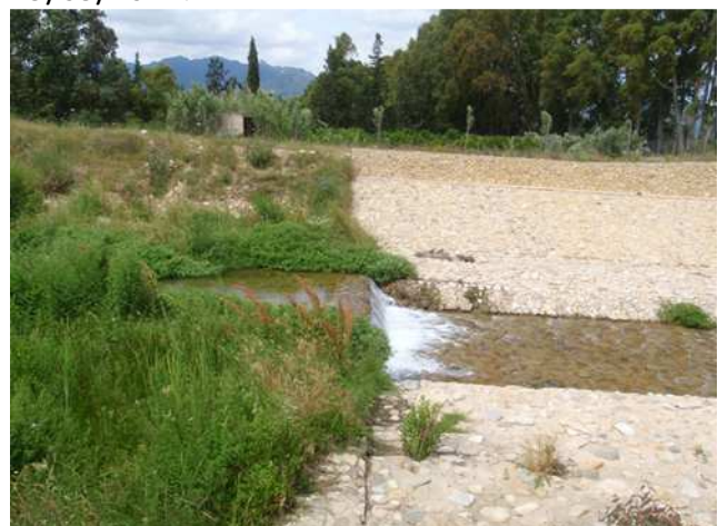
Special features/ Reinforced channel – Corr'e Pruna Monte, 19/05/2011.
