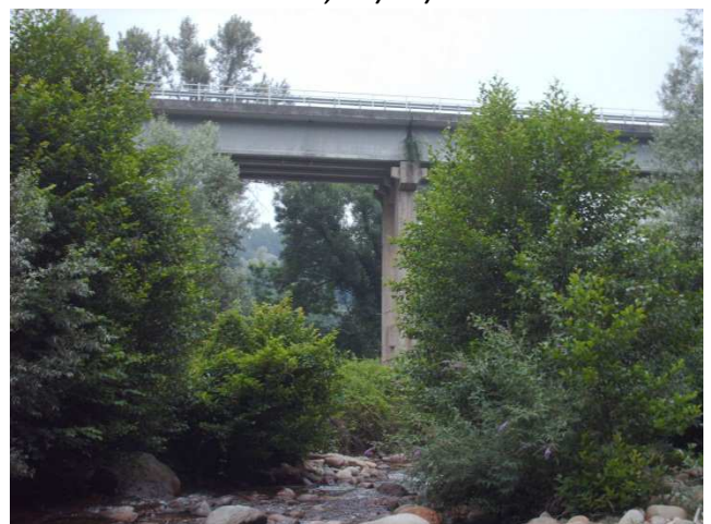
Special features/Main road bridge - Viona, 29/06/2011.
