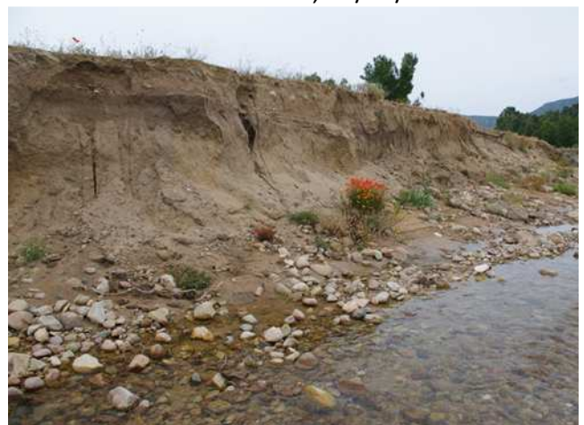
Special features/ Bank erosion - Porceddu, 21/05/2011
