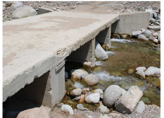
Special features/ Culvert and ford - E Gurue, 23/05/2011.
