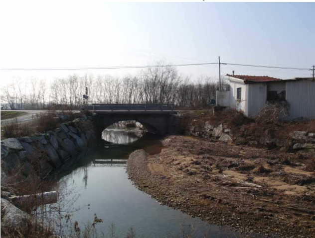
Special features/Bridge and reinforced bank - Guarabione Sdop, 24/02/2011.
