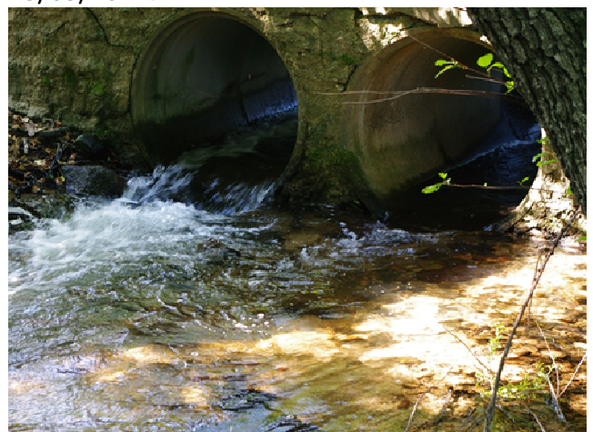
Special features/Culvert in the channel - Baldu Monte Culvert, 13/05/2011.
