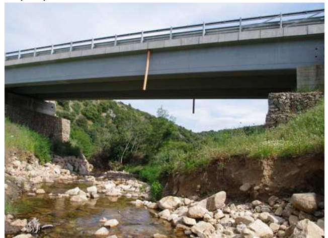
Special features/- Bridge foot in the channel - Terra Mala Valle Ponte, 14/05/2011.
