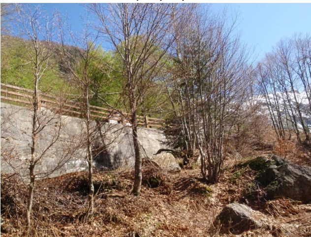
Special features/Reinforced of the road - Loana, 13/04/2011.
