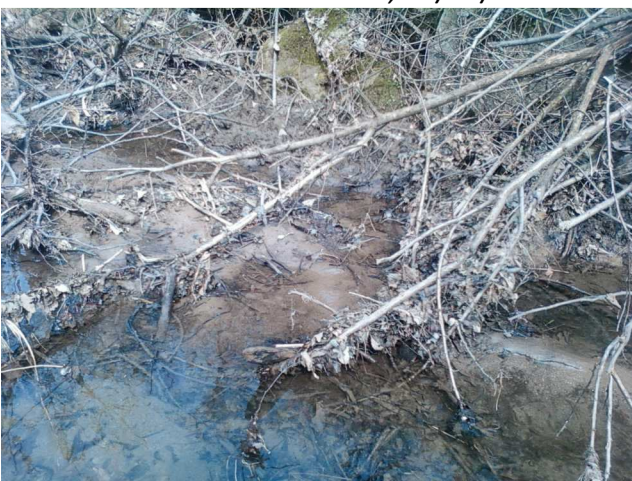
Eroding bank – Biotic habitat, 21/03/2011.
