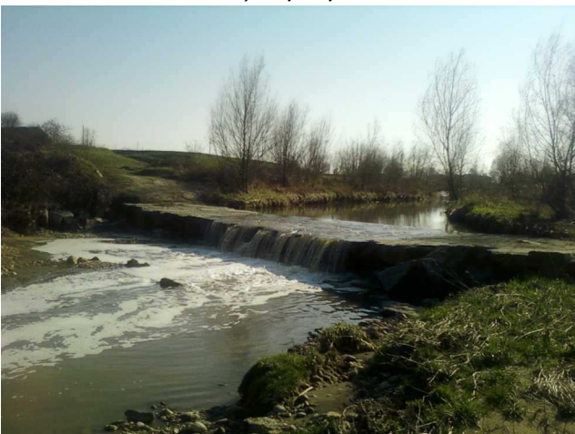
Special features/Weir - Odda, 21/03/2011.
