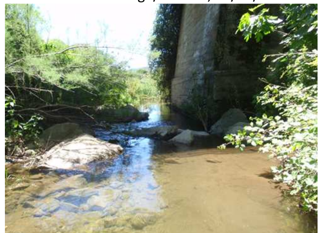
Special features/ Bridge foot in the channel - Solago/Sarossa, 17/05/2011.
