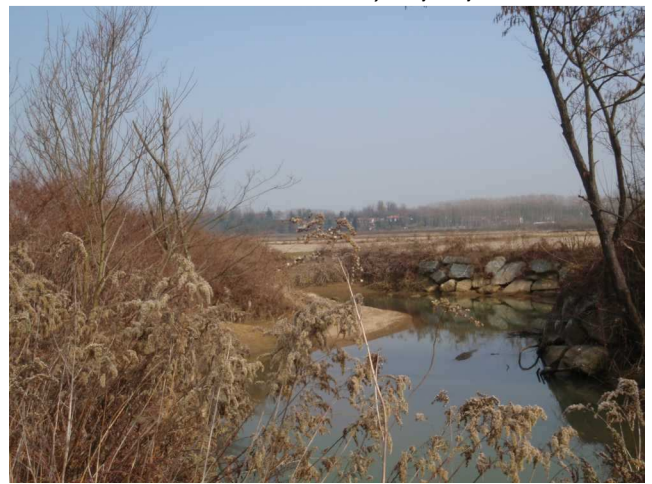
Special features/Reinforced bank - Guarabione, 24/02/2011.
