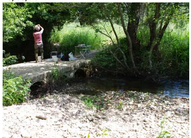
Special features/Culvert in the channel - Baldu Down Culvert, 13/05/2011.
