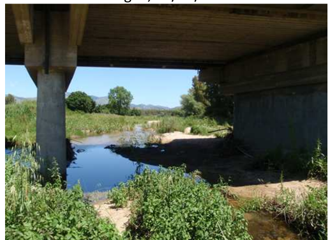
Special features/ Bridge foot in the channel and sand deposit -Irgoli, 18/05/2011.
