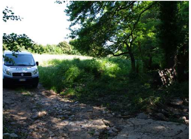
Site view/Land use - Baldu Down Culvert, 13/05/2011.
