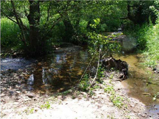
Site view/Channel – Baldu Monte Culvert, 13/05/2011.
