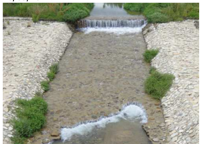
Special features/ Artificial channel armoured – Corr'e Pruna Ponte, 20/05/2011.
